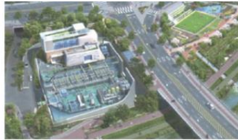
Siheung Mokgam Sewage Treatment Plant Client ----- Siheung City Capacity ----- 13,000m 3 /day
